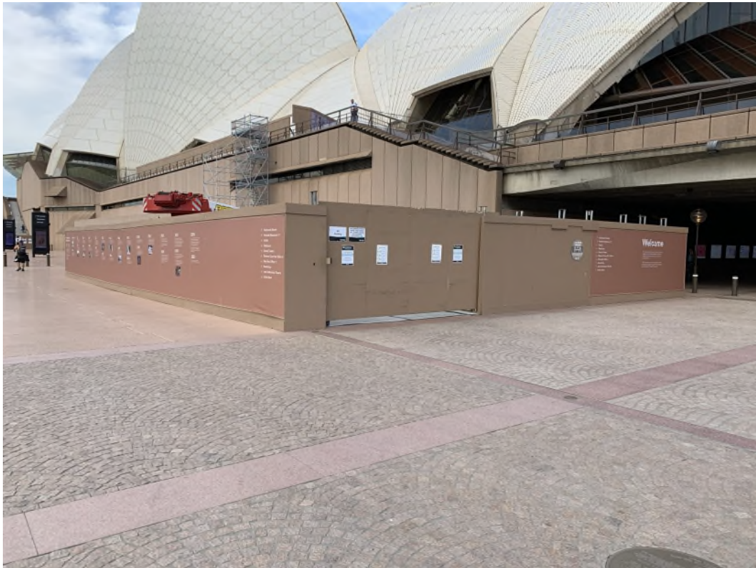
Plate 3: Hoarding around lifting zone, showing interpretation material
