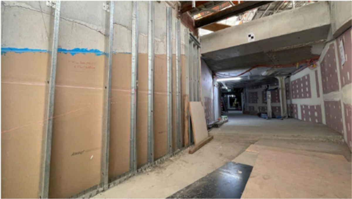
Plate 5: Construction of Eastern Passageway
