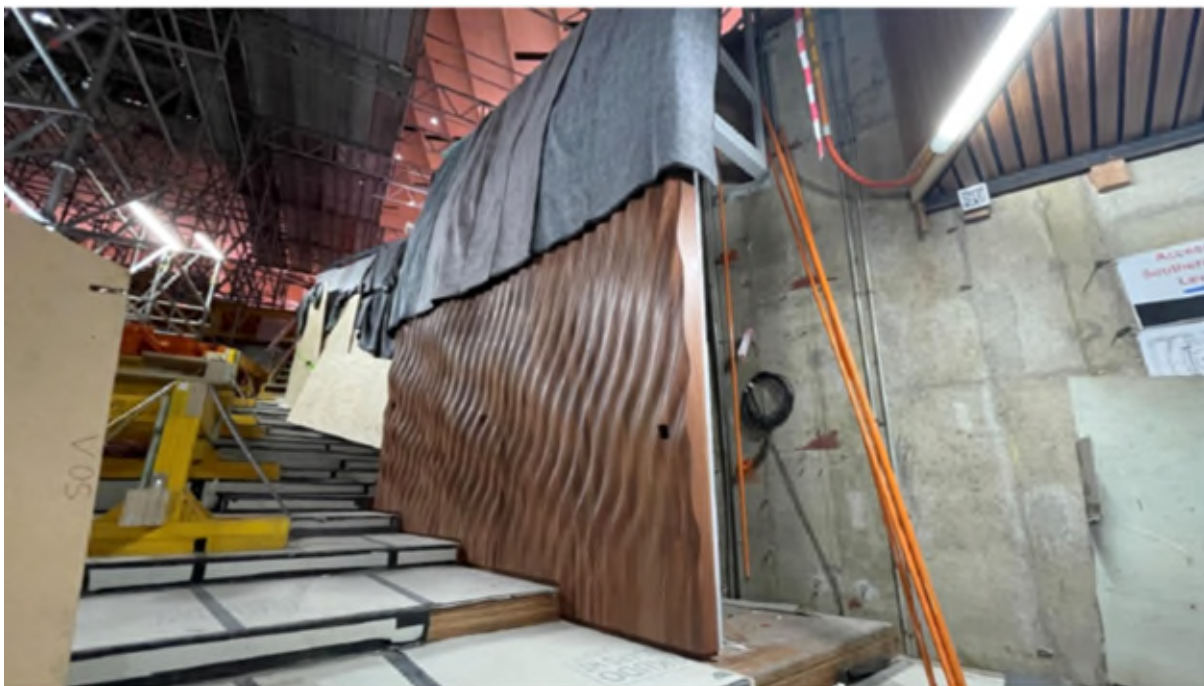
Plate 6: Diffusion Panel Installation
